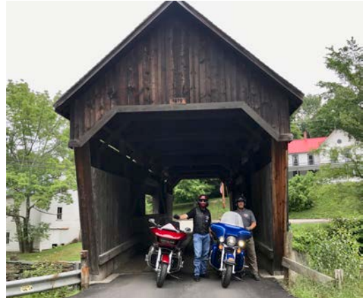
Covered Bridge on VT-100, (Bob & Steve)
